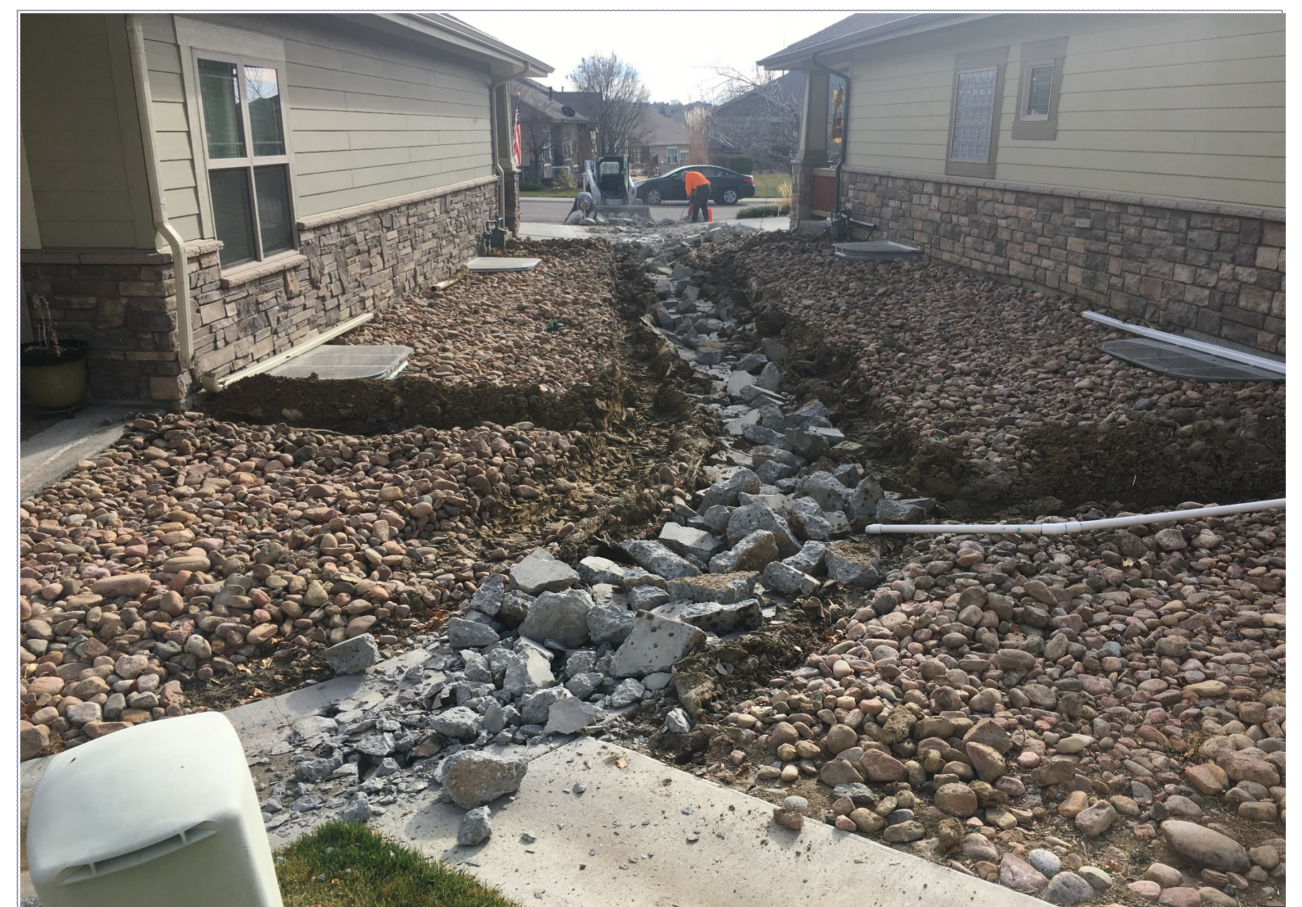
Area 7 - Demolded drain pan ready for removal
