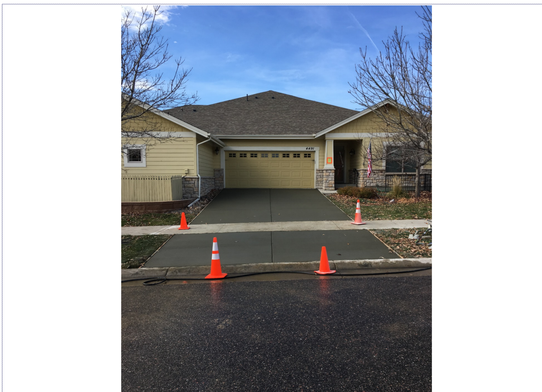
Area 16 - New drive poured
