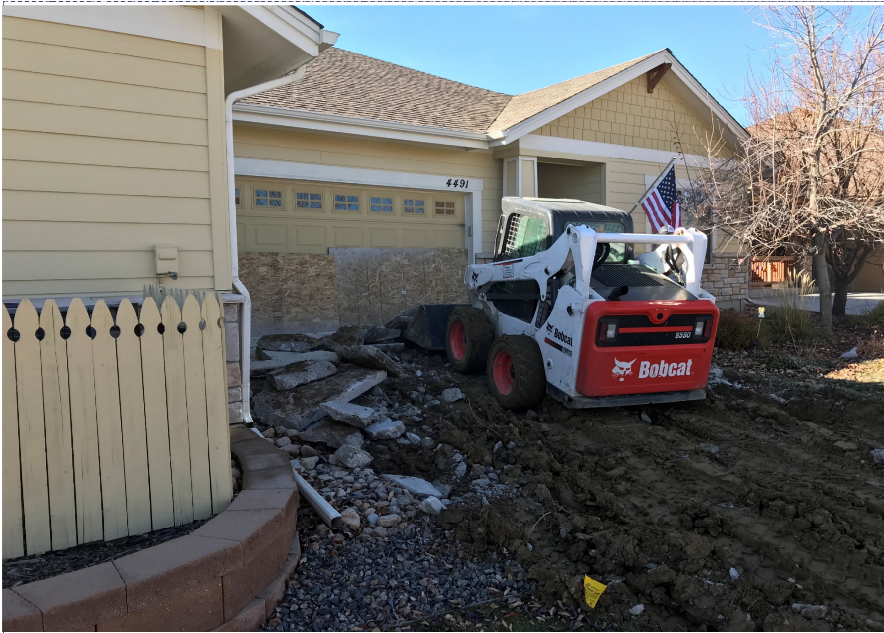
Area 16 - Crew demoing the driveway
