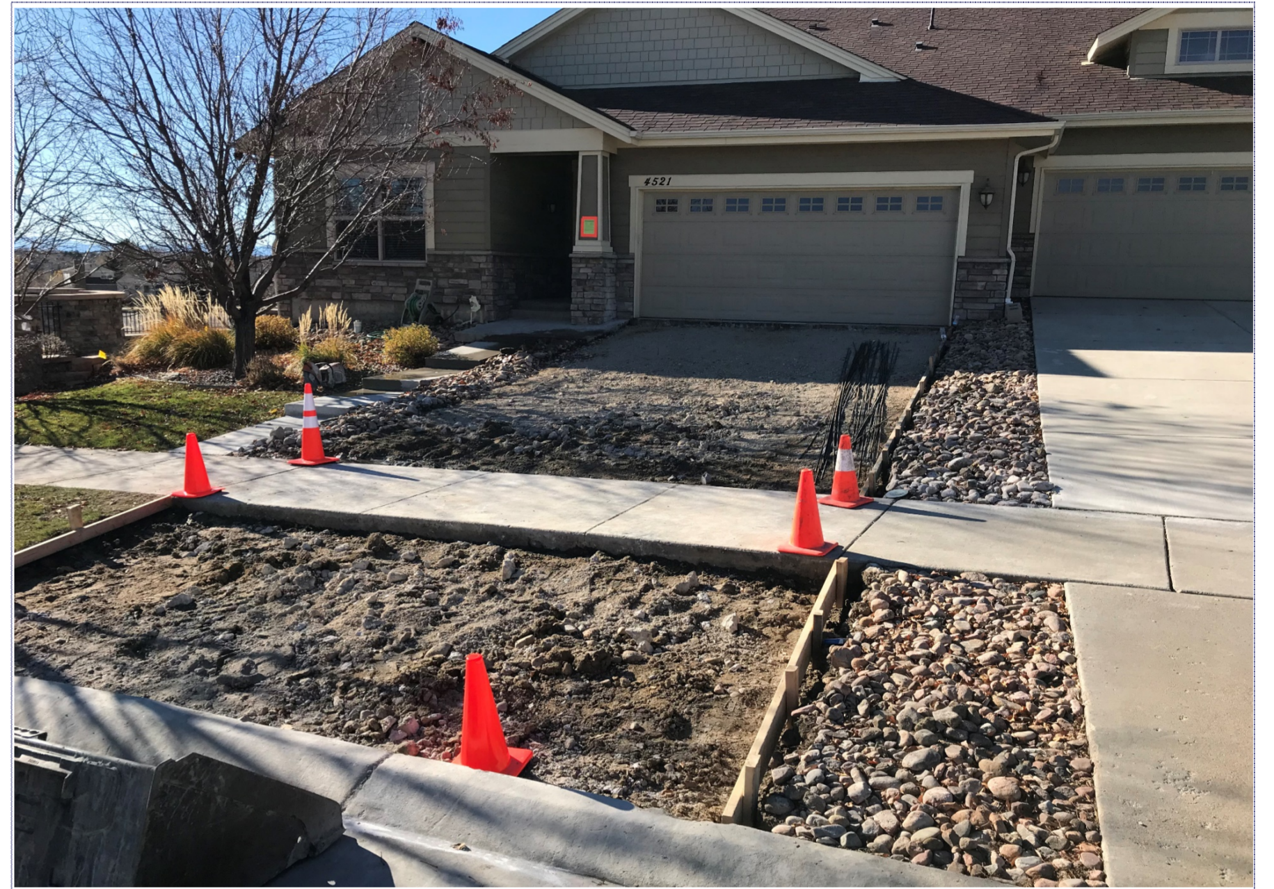
Area 17 - Fully demoed driveway.
