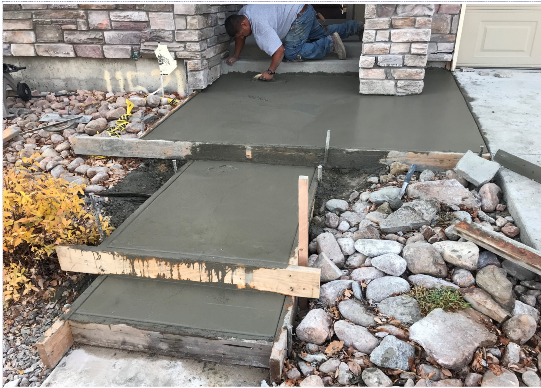
Area 17 - Change order work for the new landing and steps
