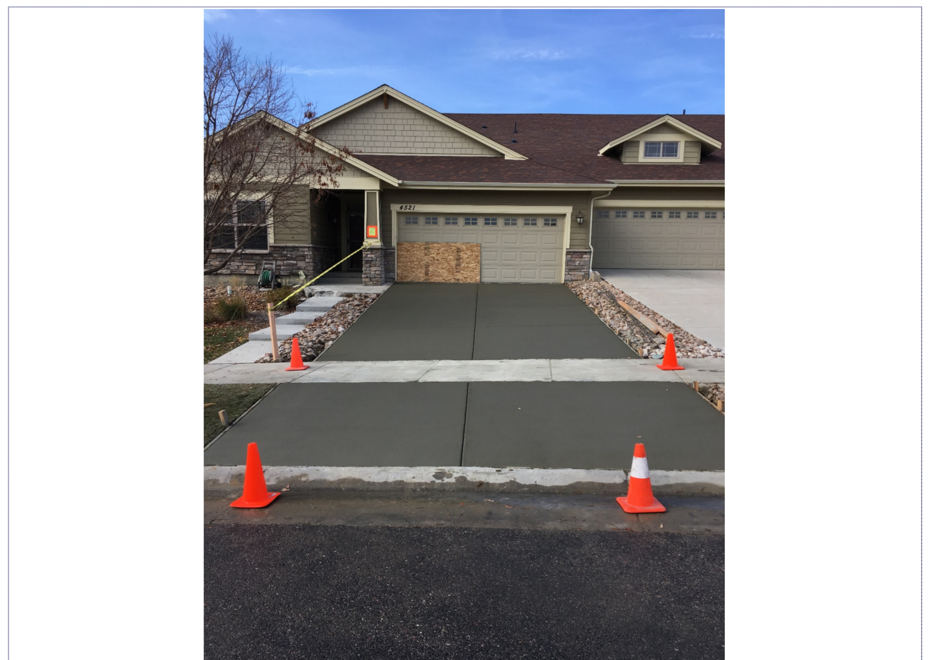
Area 17 - New drive poured
