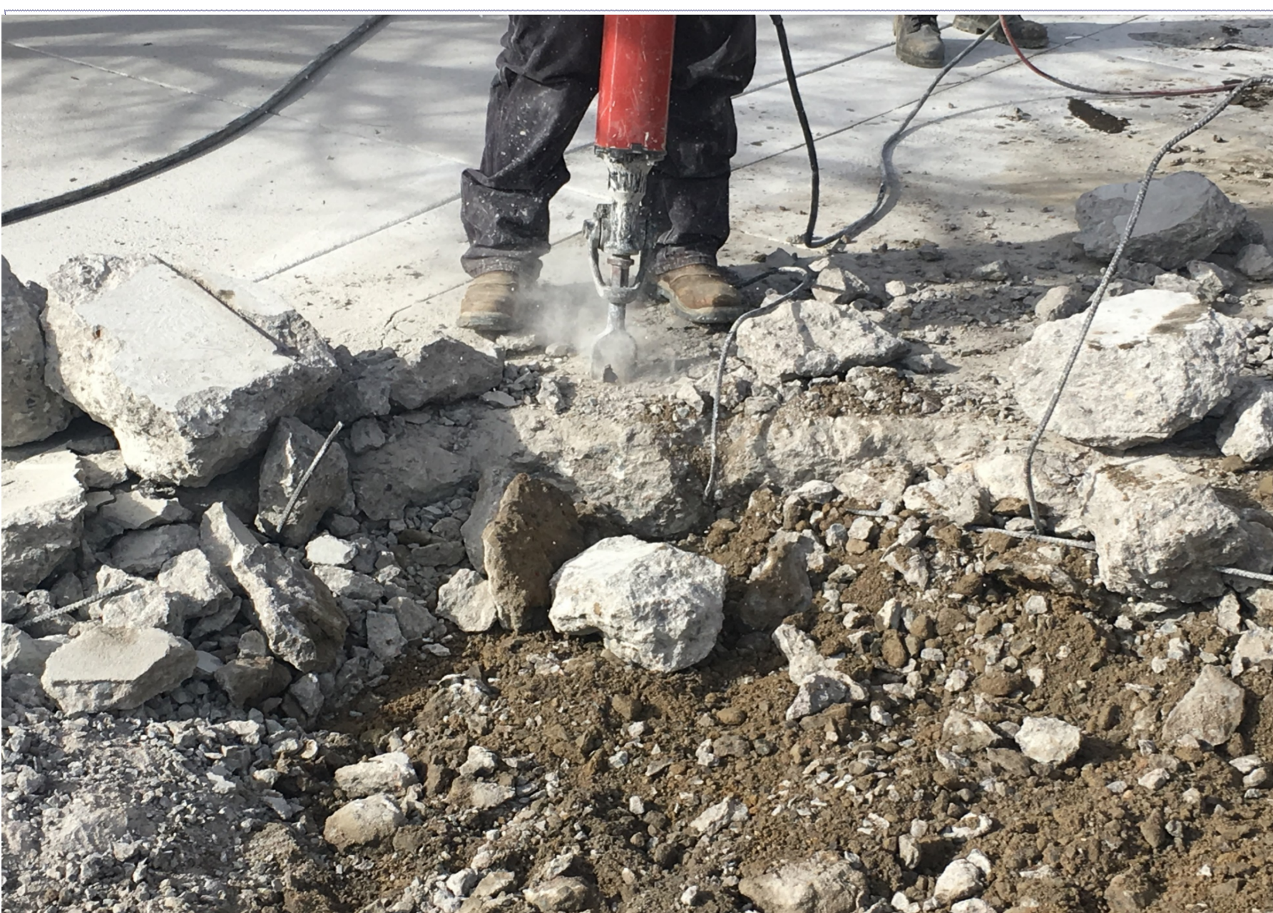
Crew member breaking up concrete
